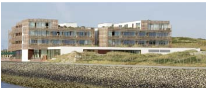
Hotel Budersand, Sylt. Hansgrohe products: Raindance Rainfall and Raindance S hand shower. Photo: jana-ebert.de
