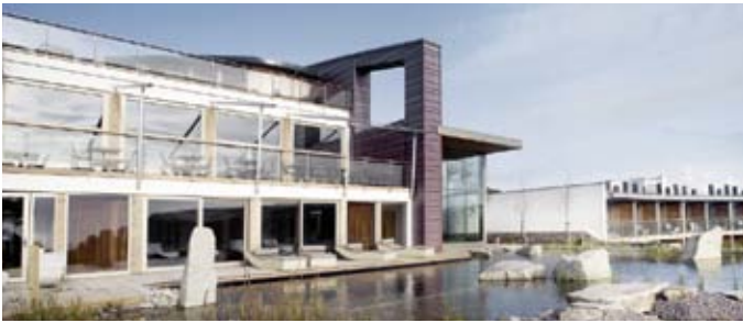
Scarlet Hotel, Cornwall. Hansgrohe products: Raindance overhead shower, Talis S basin mixer and Pontos AquaCycle 9000.
